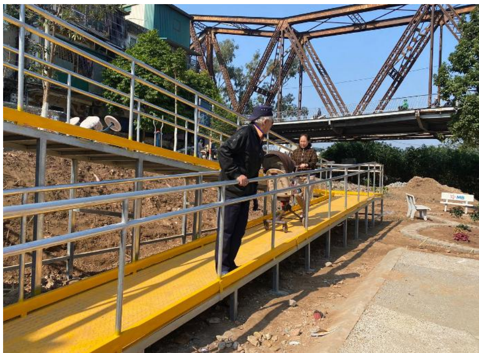
↑ Eldery using the newly installed accessibility ramp with a stroller Phúc Tân Forest Park
