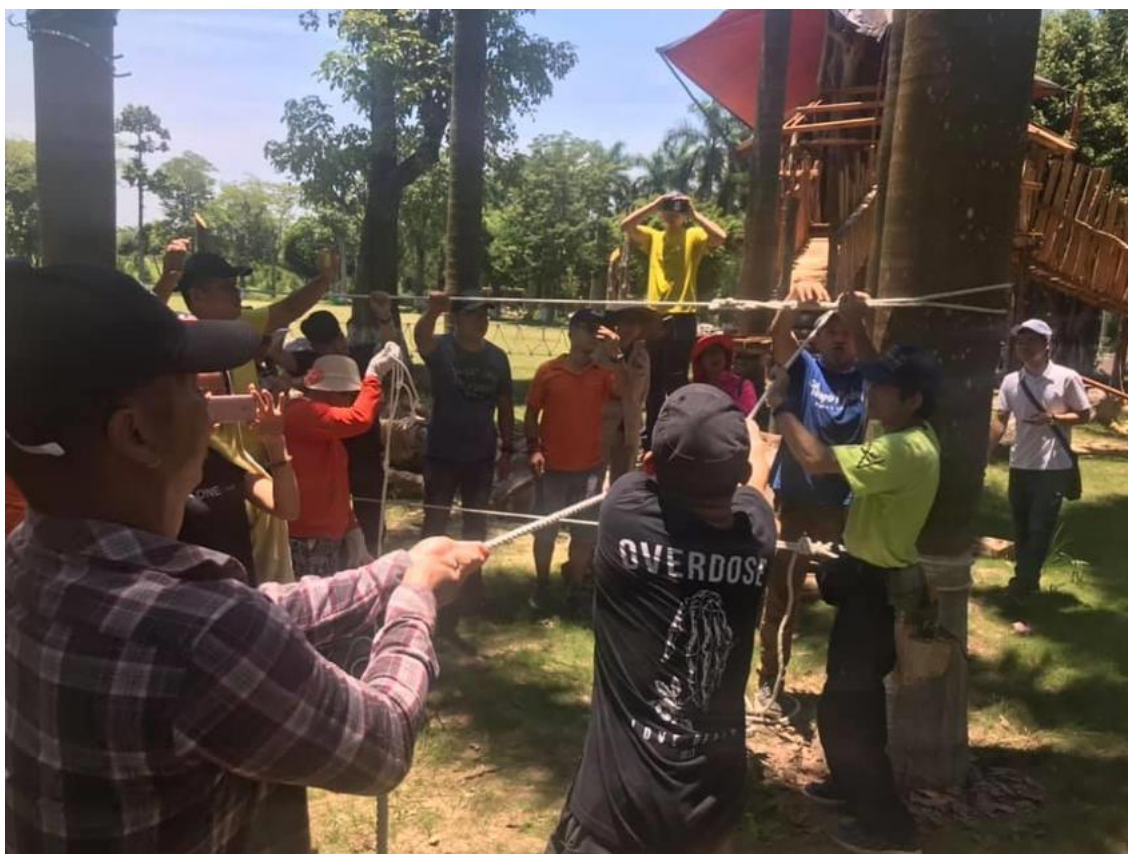
Figure 5: Building an Adventure Playground at Ecopark, 2019.
